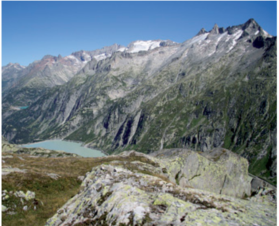
▲ View on HPP's Innertkirchen & Handeck at Rätichsbodensee
