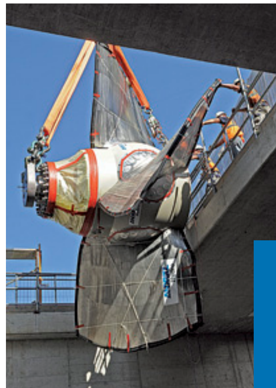
▲ Turbine runner installation
