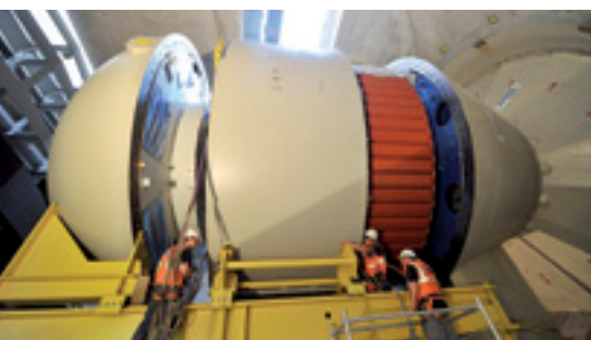
▲ Generator installation
