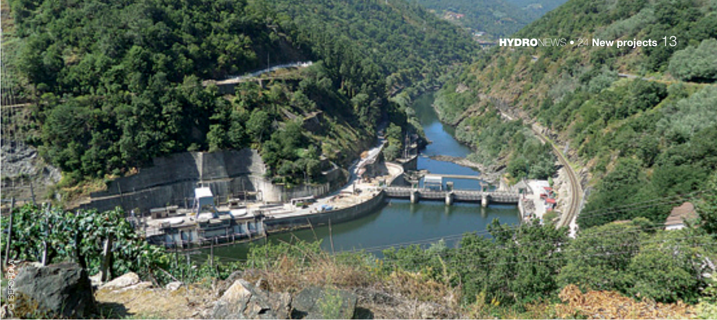
▲ View onto HPP San Pedro II from upstream
