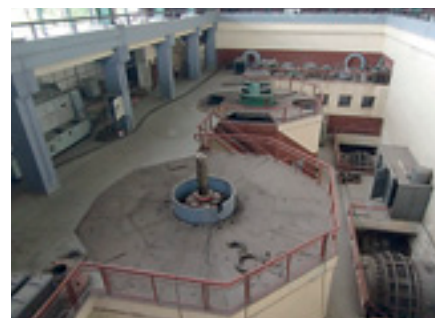
▲ HPP Djoué before rehabilitation
