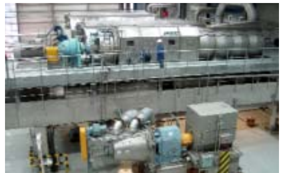
World's largest disperser and screw press at UPM-Kymmene (UK) Shotton Paper
