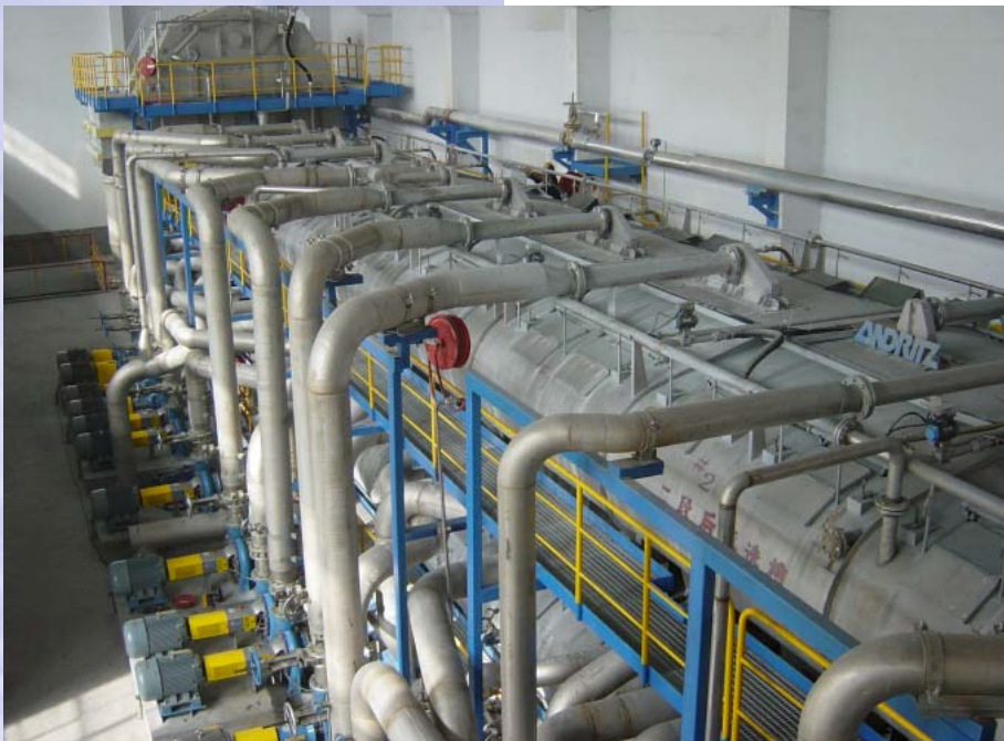
The compact design of Andritz's SelectaFlot™ flotation system was perfect for Nanping's new DIP line.
