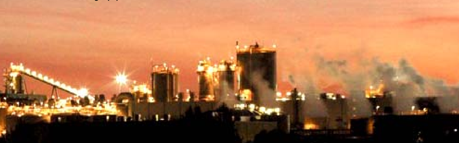
Andritz provided the major chemical recovery systems for the Stendal mill — evaporators, recovery boiler, and recausticizing equipment.
